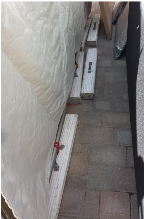
Rain gutter filled with concrete – attached to stabilizer bar
